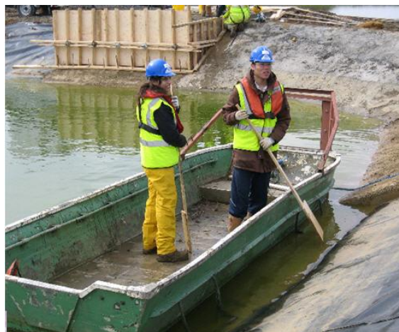
Figure 6 Working over water
