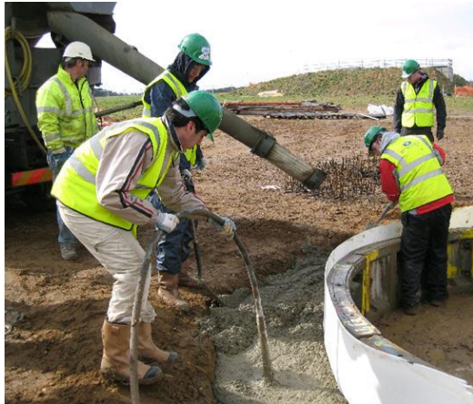
Figure 2 Constructing a concrete ground beam
