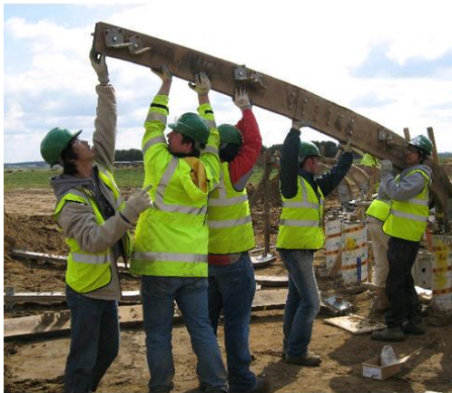
Figure 4 Lifting heavy materials
