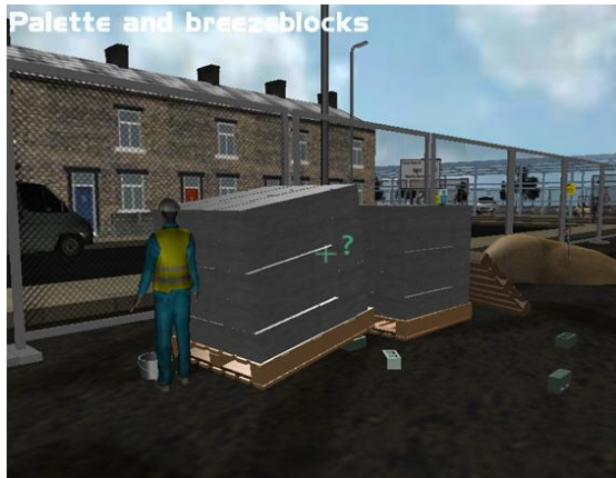
Figure 10 Incorrect storage of construction materials
