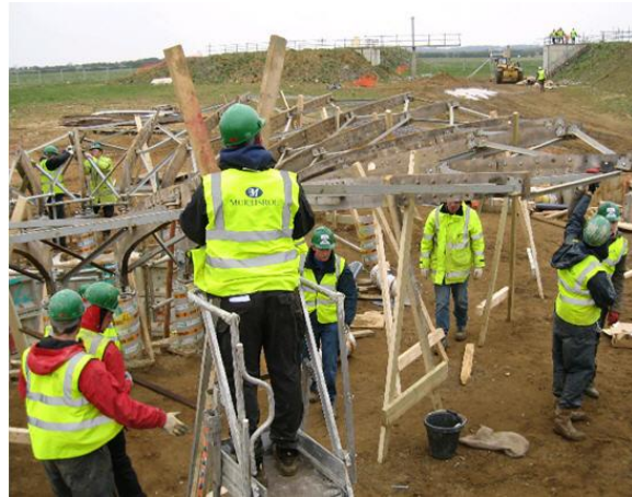
Figure 3 Working at height using a platform
