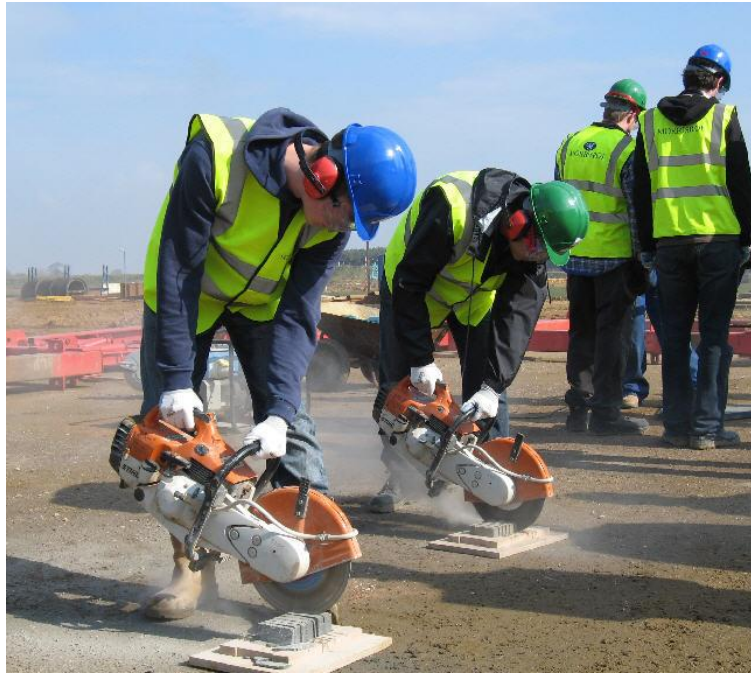
Figure 1 Constructionarium power tool training
